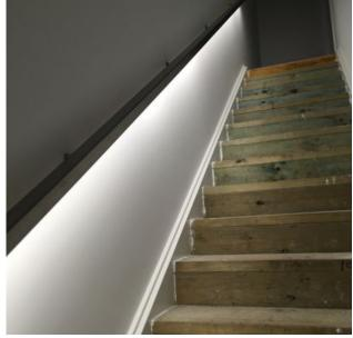
The sizes we offer LED allowances on are 50.8mm Round, 38.1mm Round & 50 x 25mm. Our handrails will come with a 15 x 15mm slot which allows for a LED channel to be installed. We will also provide holes for the wire to pass through at pre-selected points as well as run a drag wire through when installing to help with the electrical installation.
